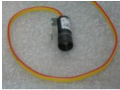
Cad Cell Eye Assembly removed from the ignitor.
