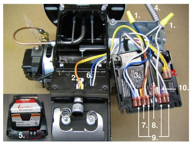
**Beckett AFG Burner to Furnace Wiring (Genisys 7505)**
