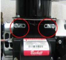
Going into the burner requires loosening of the two screws and moving the ignitor hold-downs. Lifting the ignitor will expose the oil pipe and electrodes. The copper tube (1/8”) has a hex flare nut and a splined lock nut (below) for holding the oil tube in the proper alignment.
